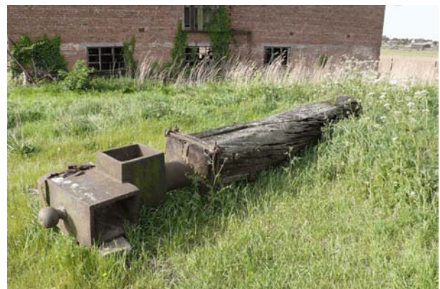
Plate 11 Windshaft and iron canister
